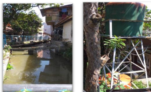
Figure 11. The private piping and torrent Source: Observation result, 2022
