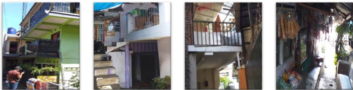
Figure 21. Vertical extension, extrusions, external stairs, add-ons Source: Observation result, 2022
